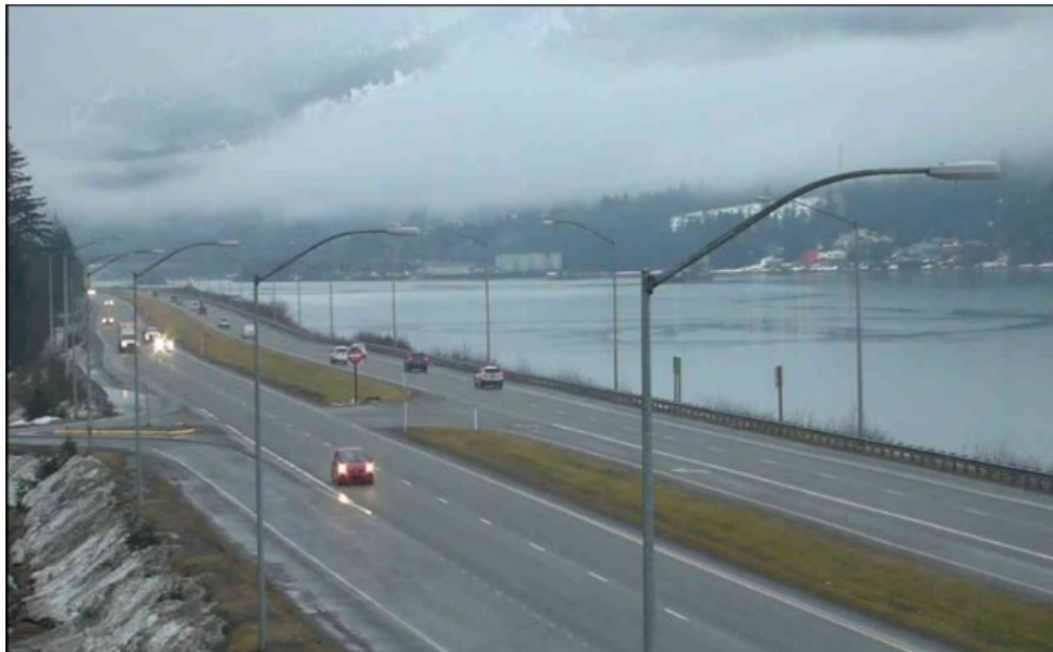
Figure 18: RWIS Station at Milepost 3, Egan Highway (Retrieved January 15, 2026, DOT&PF Winter Operations Dashboard)
